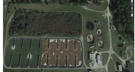
Alex City Sugar Creek WWTP
